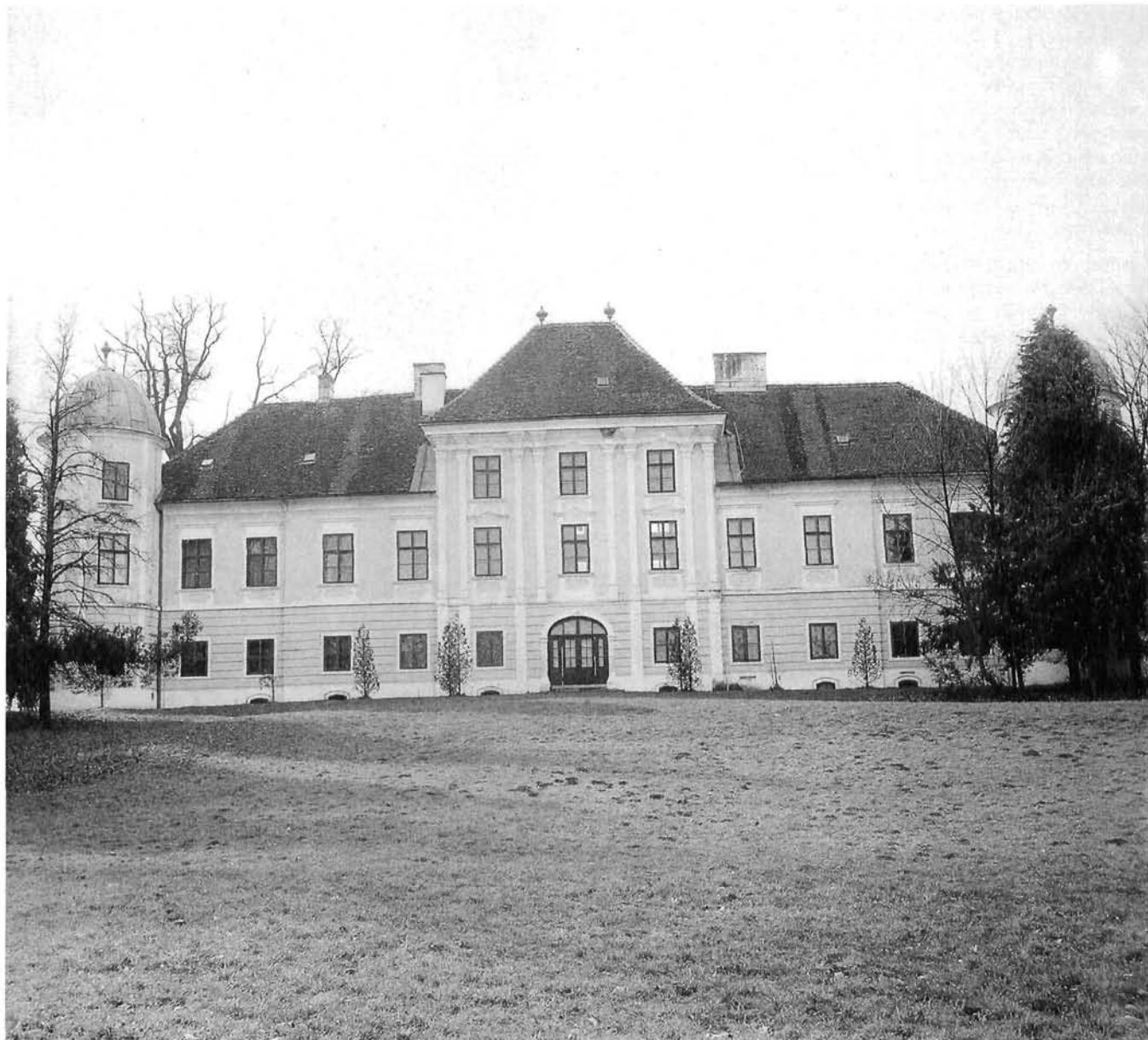
Dvorac Brezovica, pročelje Brezovica castle, the facade
