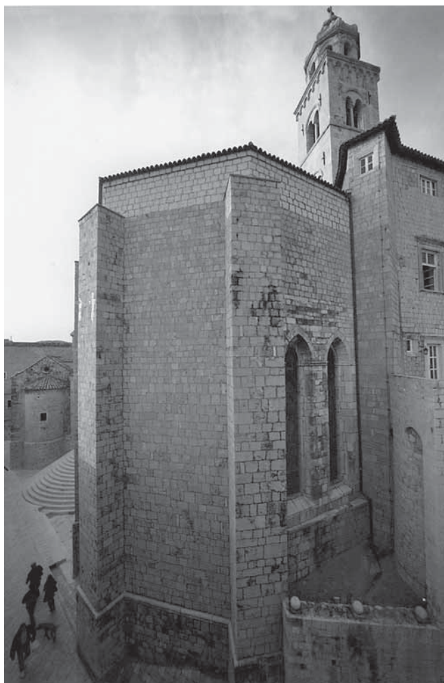
4. Dubrovnik, Crkva sv. Dominika, začelje, pogled s jugoistoka Dubrovnik, Church of St Dominic, exterior of the apse from southeast
