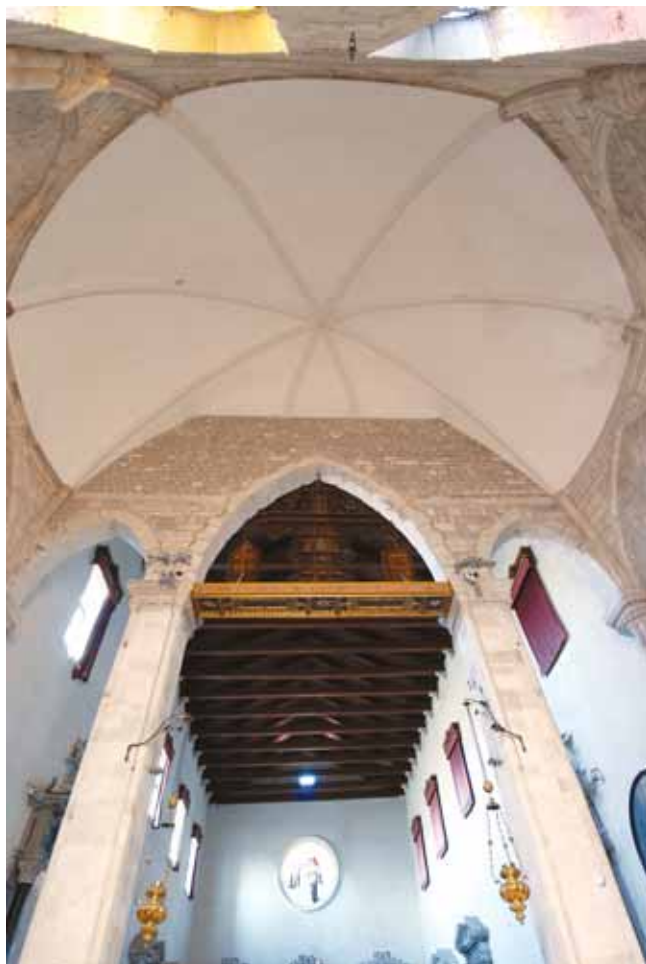
7. Dubrovnik, Crkva sv. Dominika, svod apside Dubrovnik, Church of St Dominic, apsidal vaulting
