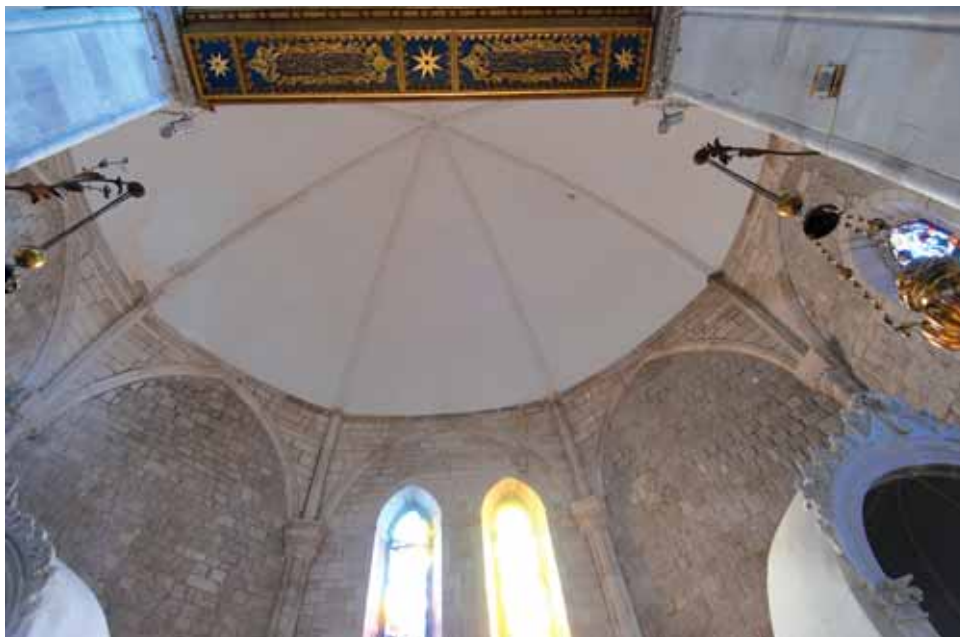
5. Dubrovnik, Crkva sv. Dominika, konstrukcija apsida Dubrovnik, Church of St Dominic, the construction of the apse
