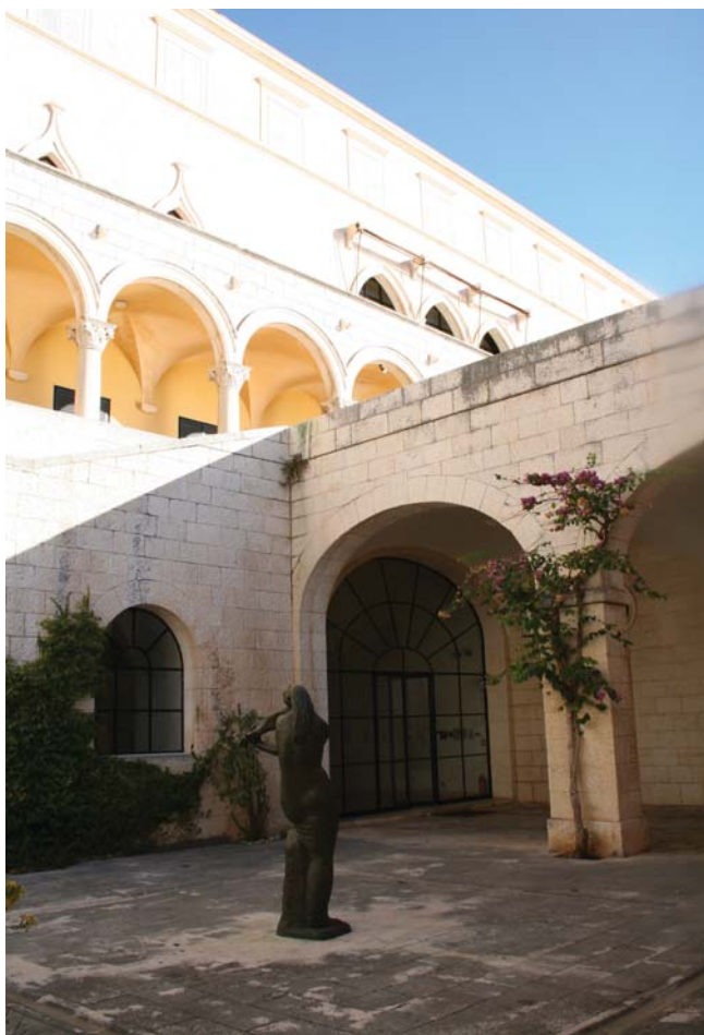
7. Palača B. Banac na Pločama u Dubrovniku, Put Frana Supila 23, peristil, 2008. Palace of B. Banac at Ploče in Dubrovnik, Frana Supila St. No. 23, peristyle, 2008
